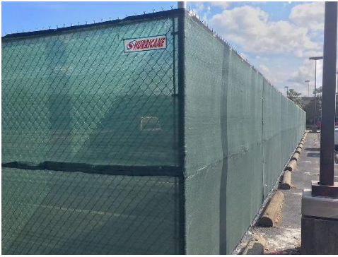
Example of a temporary construction fence
